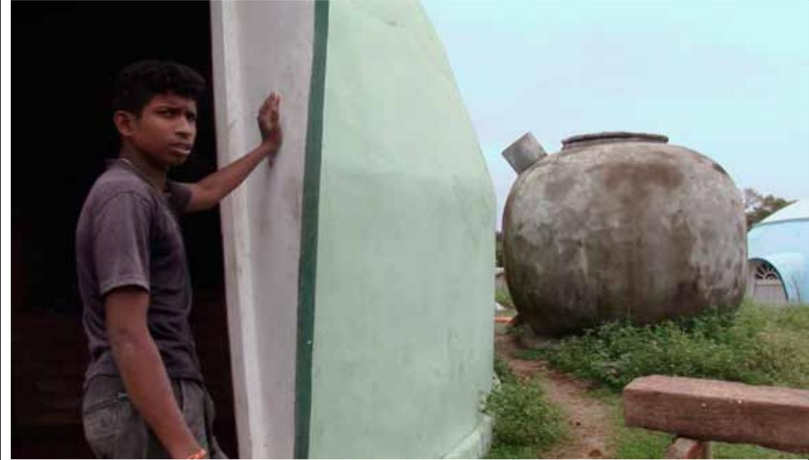
The igloo structures were built by pouring concrete over an inflatable hull. They are designed to withstand future tsunamis. The houses have kitchens with a traditional open fireplace, two bedrooms and a living room; there are teapot-shaped water collection tanks and eco-toilets outside.
